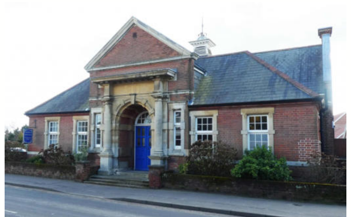
The old courthouse, now a community centre, Yarmouth Road, Blofield. 2020.
